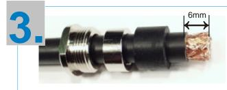
Remove 6 mm of the PVC sheath from the end of the cable with a knife.
